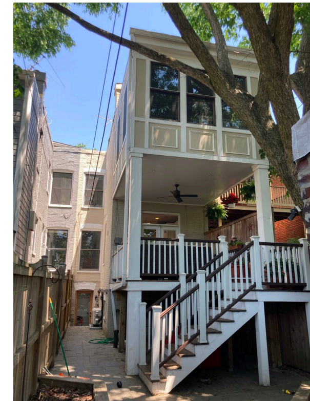
EXISTING REAR FACADE
