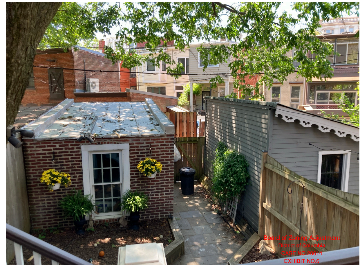
EXISTING REAR YARD
